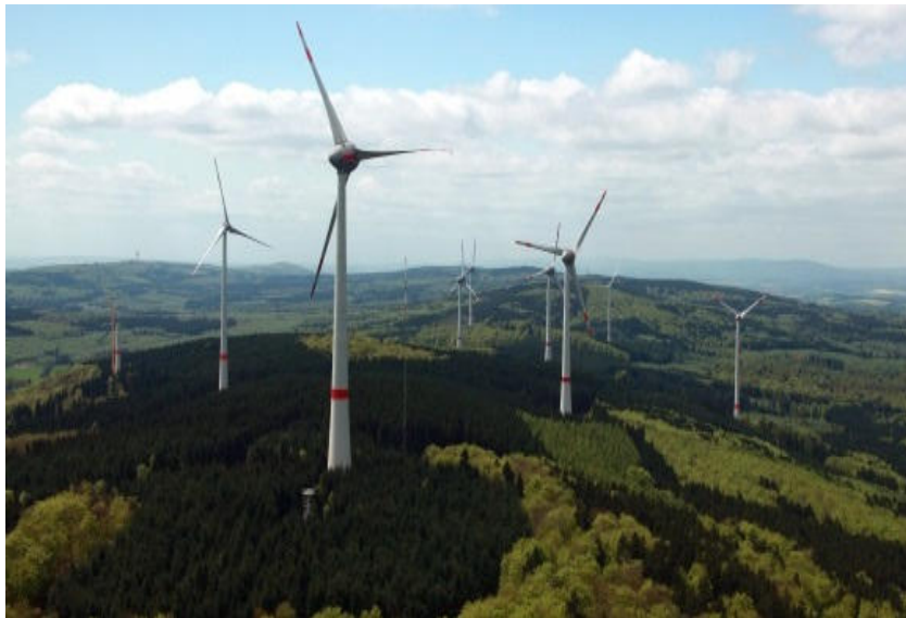
Windpark Soonwald, RLP (70,5 MW)
